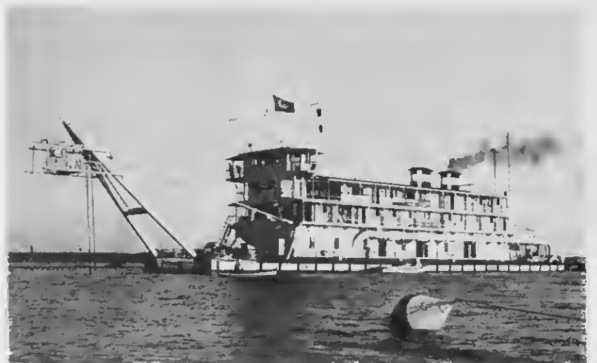
DREDGES LIKE this one keep the canal at a proper and safe depth. One of the big problems is the drifting, blowing sand, which could clog the channel unless there was constant maintenance.
